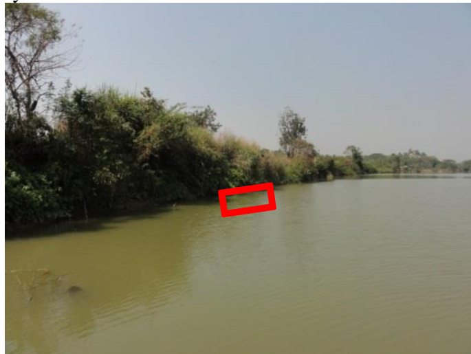
Figure 5-11: Location of the floating water pump (February 2017)
