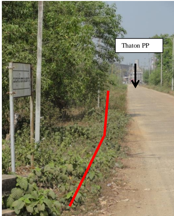
Figure 5-18: The water pipeline leaving the PP will run strictly parallel to the existing asphalted road
