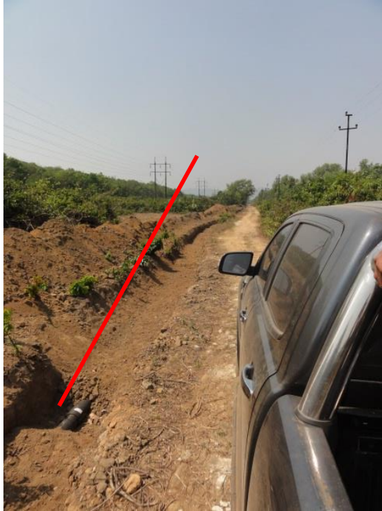
Figure 5-2: Water pipeline running parallel to the track partly finished (February 2017)
