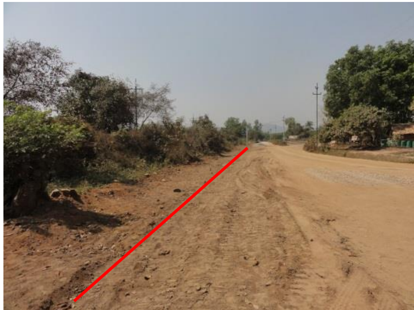
Figure 5-3: Water pipeline running parallel to the track finished (February 2017)
