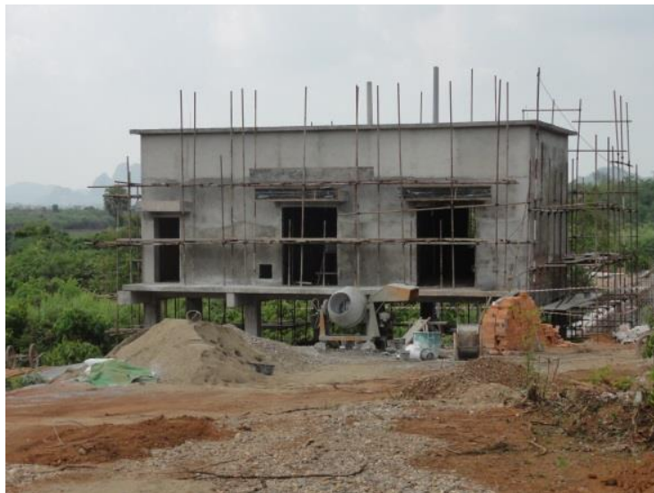
Figure 5-16: Control building (May 2017)
