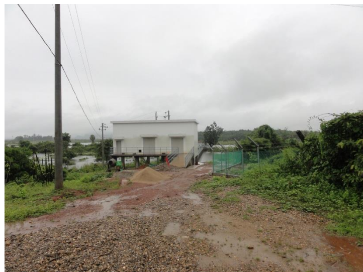
Figure 5-17: Control building (August 2017)
