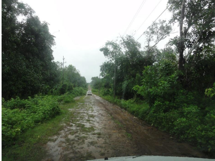
Figure 5-4: Track to pumping station with new OHL (right side). The trench of the water pipeline is just barely visible (August 2017)
