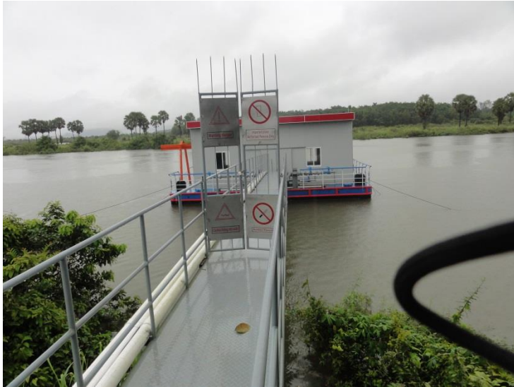
Figure 5-15: Pumping station with blocked and locked entrance (August 2017)
